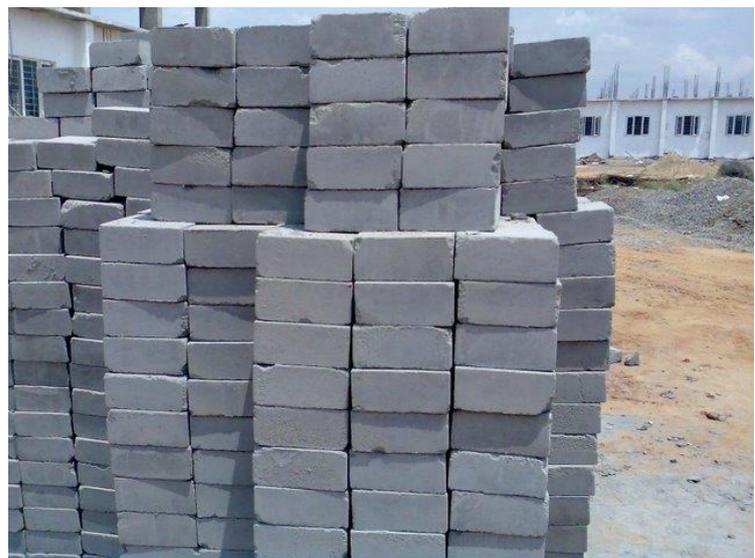
Figure 1: Fly Ash Bricks. Engineers Daily 2018
