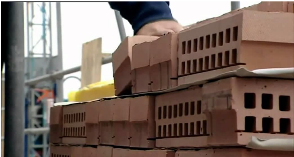
Figure 2: Bricks are shaped to interlock
